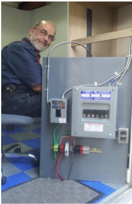
John KF7ZWX installing Electrical
