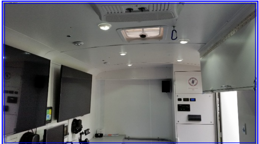
ARES Trailer Progress Interior
